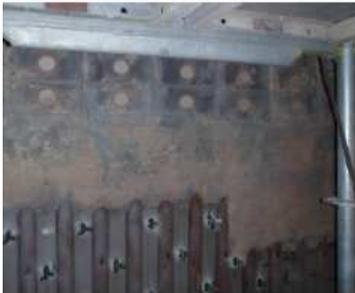
Fig 13: Corroded tubes after refractory boundary
