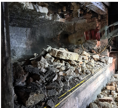
The 25-ton aluminum melting furnace during the wrecking of the old refractory lining.
