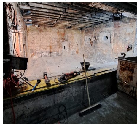
The 25-ton aluminum melting furnace during the wrecking of the old refractory lining.
