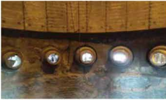
Figure 5: Lining condition before Shotcrete
