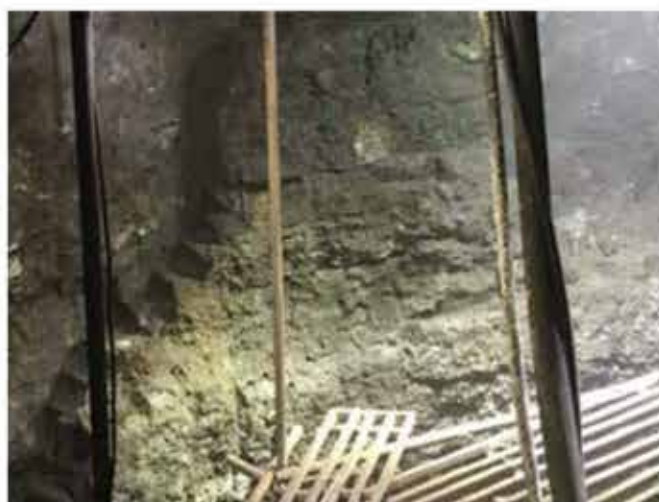
Figure 4: View of the old lining
