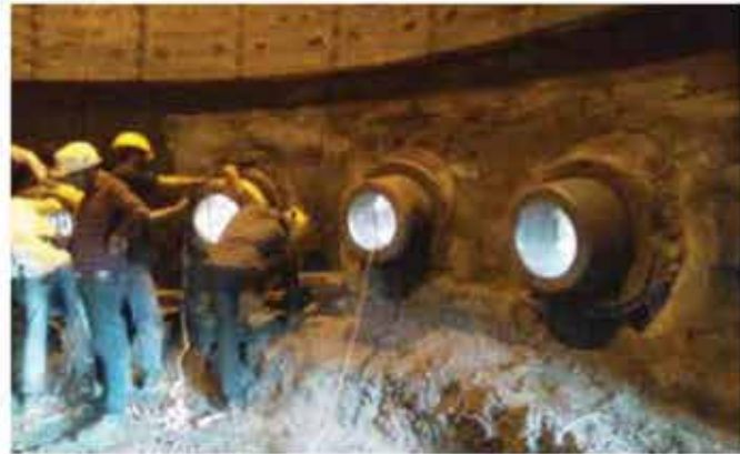
Figure 13: Lining before Shotcrete
