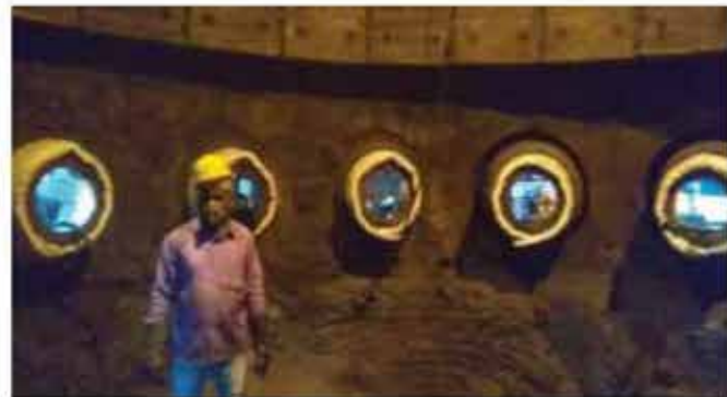
Figure 14: Preparation of the Shotcrete
