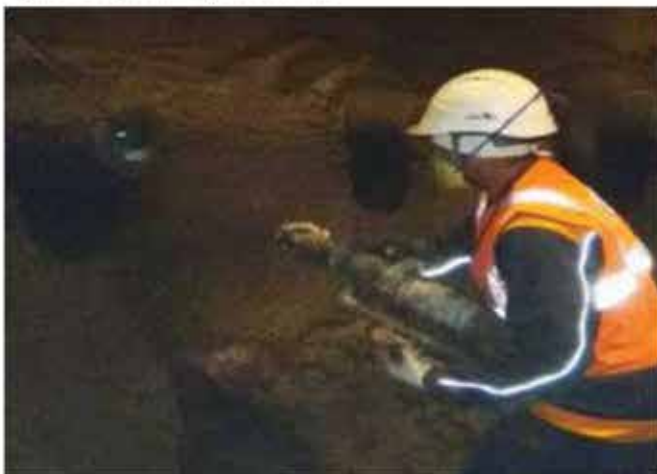
Figure 7: Installation of Shotcrete
