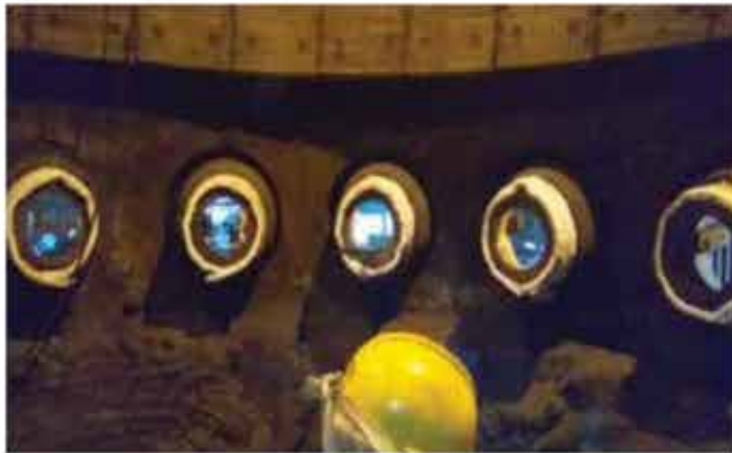
Figure 6: Preparation of the Shotcrete
