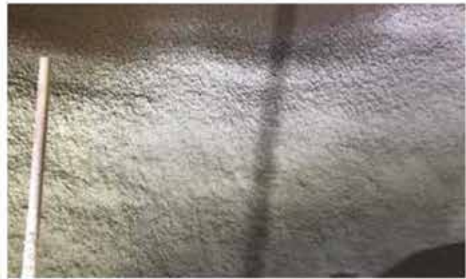
Figure 9: Lining condition after Shotcrete
